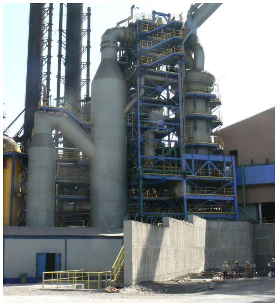
Figure 2: Gas Cleaning Plant AHMSA BF 6, 2010
