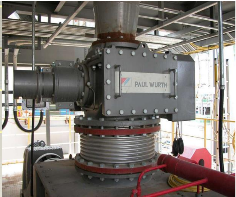
Figure 6: PW GRITZKO Valve for dust discharge
